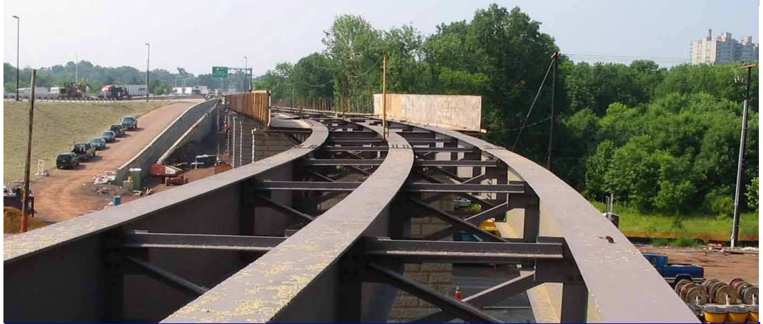
Multi-use Path No. 1 over River Road Bridge
