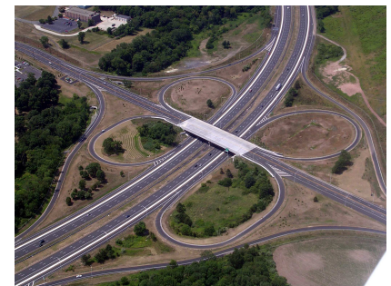
Aerial of completed interchange
