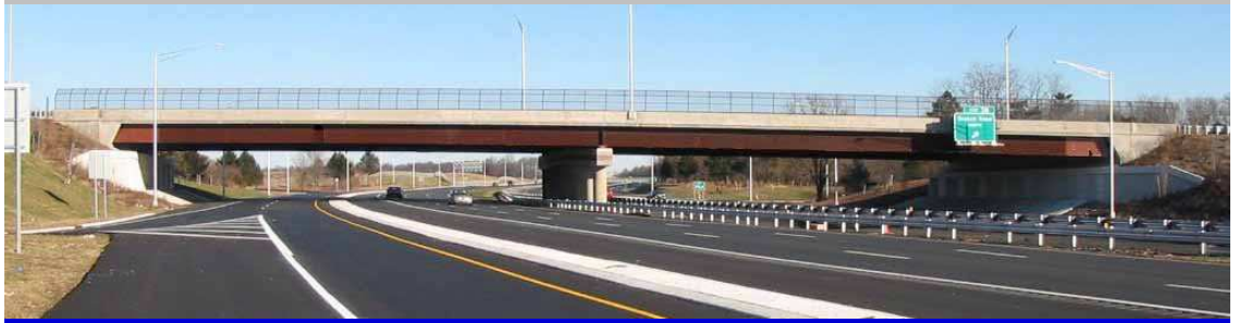
Scotch Road (CR 611) over Interstate 95
