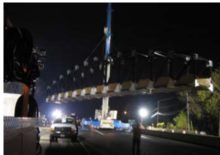
Arora designed the structure for a single lifting operation.
