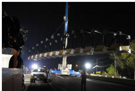
The preassembled main span truss is lifted into place.
