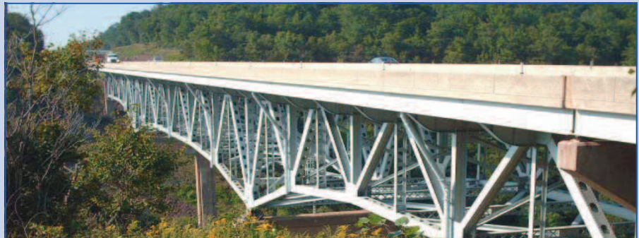
The Hawk Falls Bridge over Mud Run
