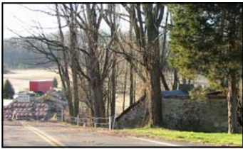
Lower Saucon Road Bridge (left) was washed out during flooding from Hurricane Ivan. Building (right) is part of the historic Pichel Farm adding an archaeological challenge to the project.
