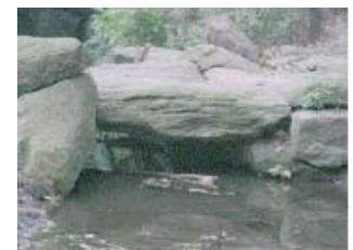
A Rock Slab Pedestrian Bridge
